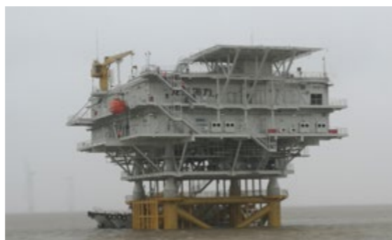
Jiangjiasha Offshore Booster Station.
