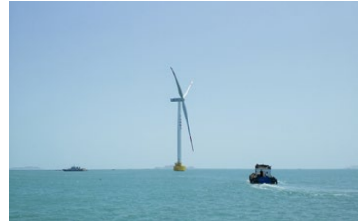
Longyuan Fujian Company Wind Farm.
