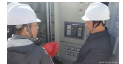
On October 24, 2018, Longyuan Safety Supervision Department went to the Longyuan Shanxi Shuangjing Wind Farm to carry out the autumn safety inspection.
